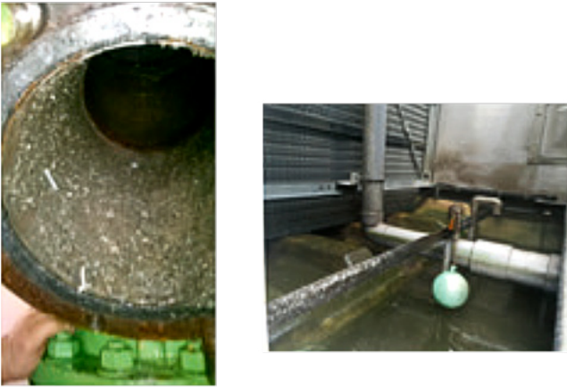
Picture 2: Biofilm growth at the pipes and the reservoir of the cooling tower
