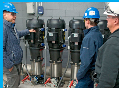
Top: The expanded range of Grundfos CRs allows the highly reliable vertical multistage pump to be used in a broader range of applications.
