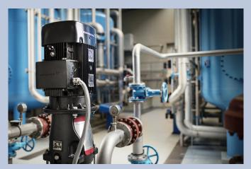
Image: The Grundfos CR-95 multistage pump at WVSB in Oberwart, Austria. The pump was much smaller than the other, older pumps from a different brand in the boosting/filtration application.
