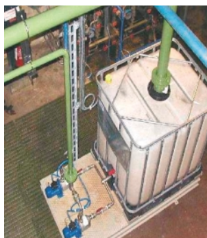
recirculation of process water
